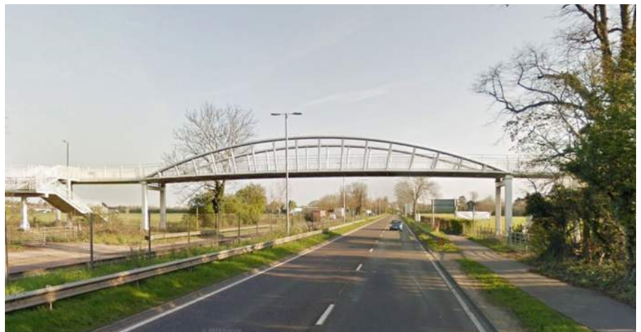
Active travel bridge over the A10 in Cheshunt (©Google).
