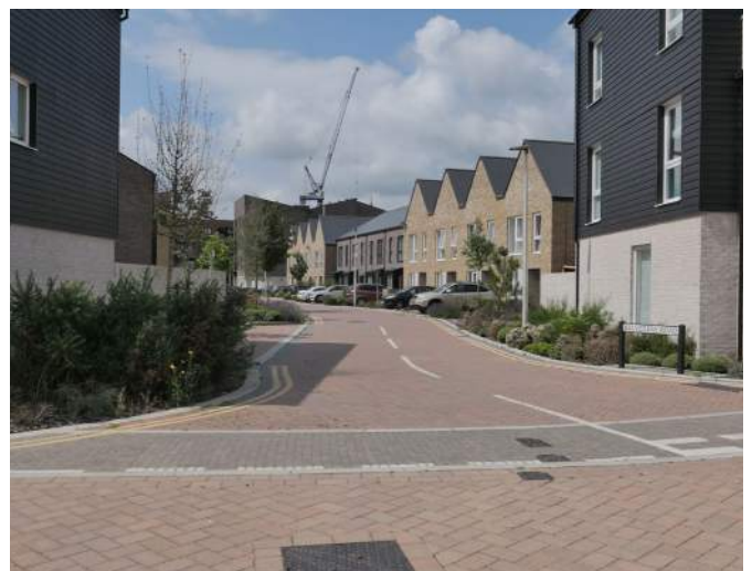
Traffic Calming Measures
