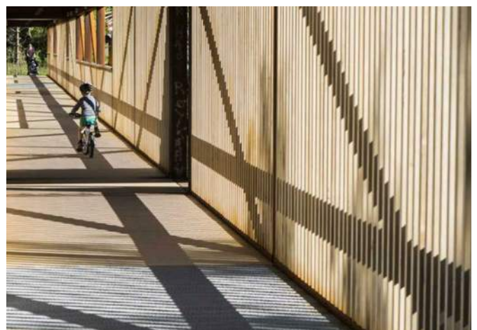
Active Travel Bridge in Norway (© Rintala Eggertsson Architects).
