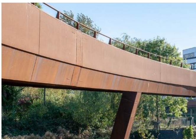
Active Travel Bridge in Northampton.
